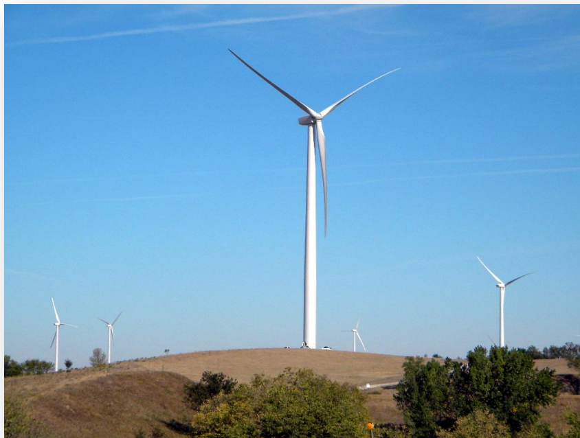
Broken Bow Nebraska Wind Facility
