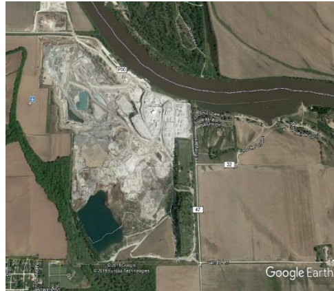
An Aerial of a Mining and Mineral Extraction Site and Quarry Source: Google Earth
