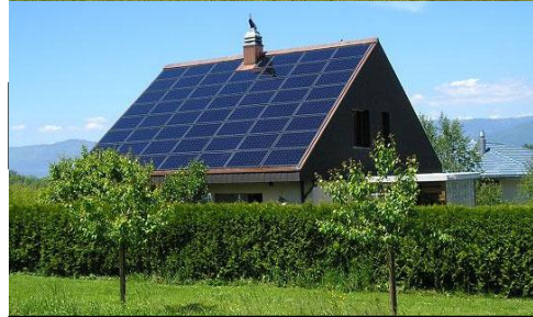
Example of a Solar Conversion System, Structure-mounted
